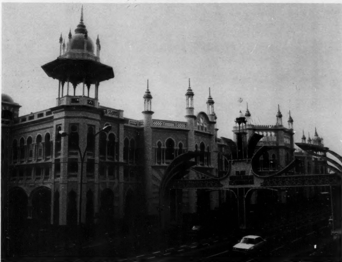
The Kuala Lumpur train station.
